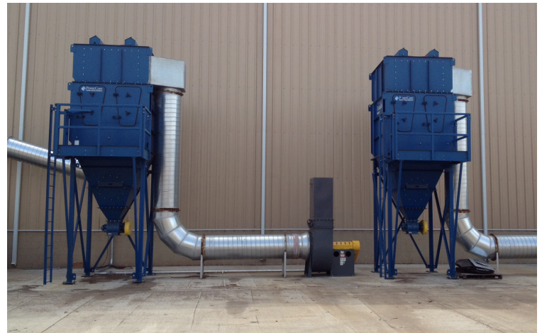
VH 2-12 on Pipe Grinding
