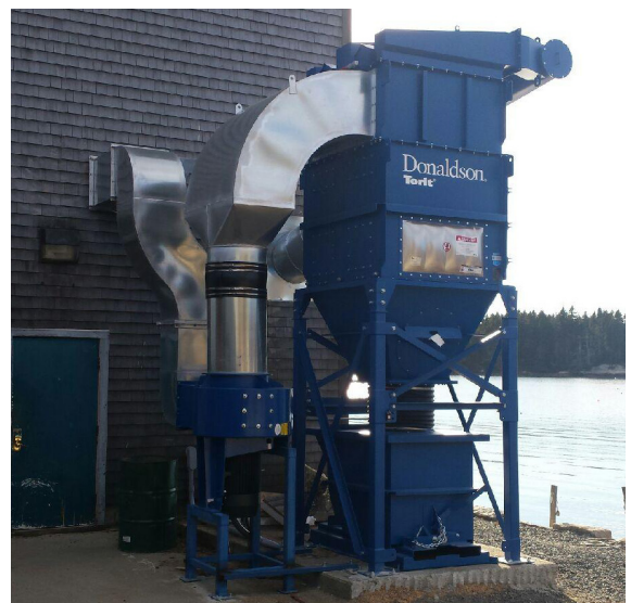
POWERCORE® VL 2-8 on Wood Dust 10,000 cfm (16,987 m 3 /h)
