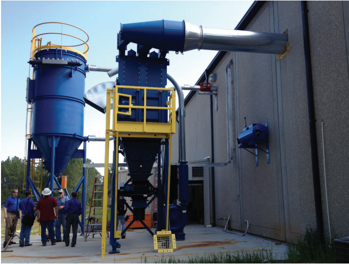
POWERCORE® VL 2-12 on Super Absorbent Polymer 14,500 cfm (24,630 m 3 /h)
