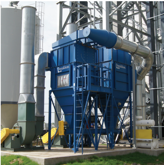
POWERCORE® VL 2-12 on Grain Dump 14,700 cfm (24,970 m 3 /h)
